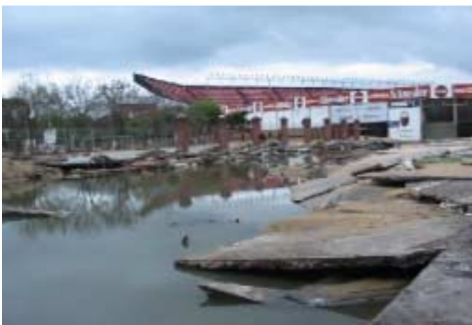
Figure 5: Flood aftermath at the soccer stadium of Colón de Santa Fe.
